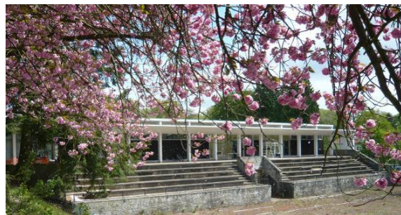
New office space in the sports center- front view of the renovated 'D Building'
